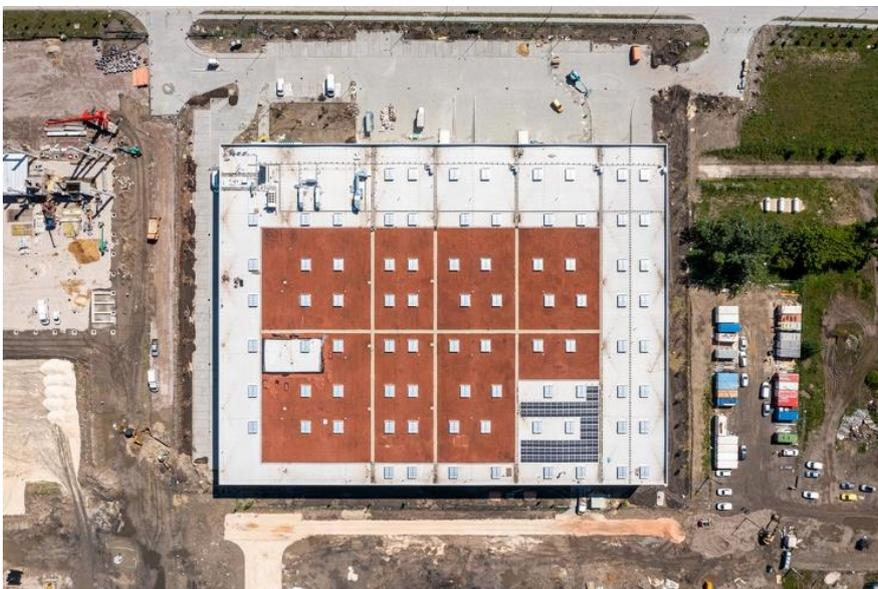
Picture 2: 10% sun panels and 60% green roof (the red parts) will cover the new “D3” building in the Freeport of Budapest (photo was taken on the 7/6/2021)
