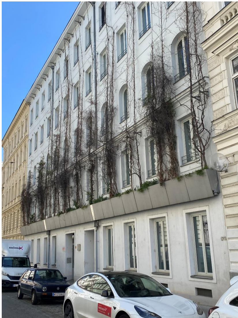
Picture 2: Greening from the 1 st floor (Embelgasse, B)
