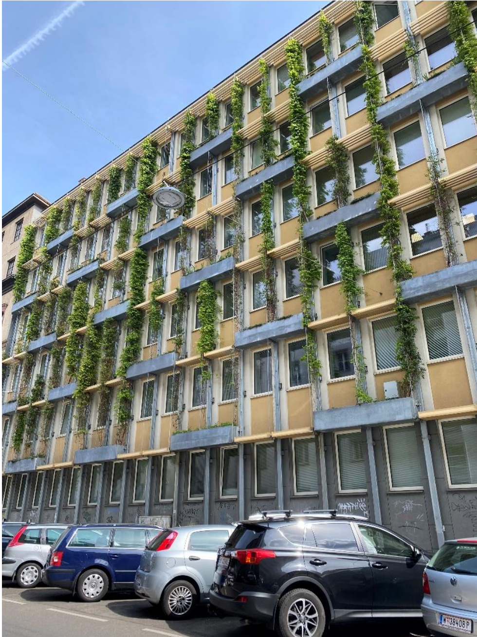
Picture 4: Steel-structure for the plants (Grabnergasse 4. E)
