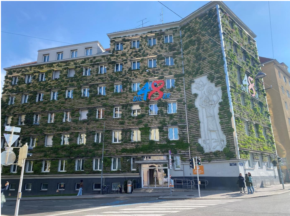
Picture 7: - Green wall of the waste management company (Einsiedlergasse 2. A)
