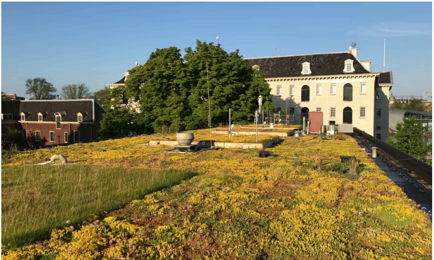
The blue-green roof functions like 'a flat rain barrel'. Photograph: Resilio
