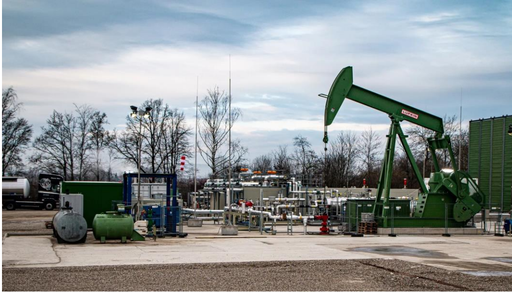
Infrastructure for testing the Ampfing oil deposit (Bavaria)
