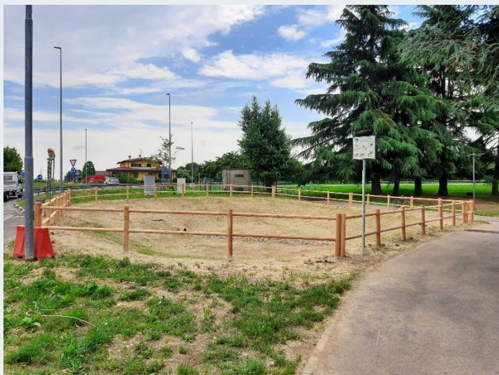
Figure 4. Detention pond constructed in the Municipality of Masate
