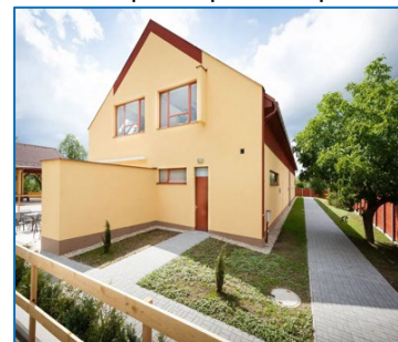
Photo 3 - paved path to apartments
