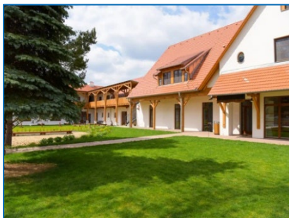
Photo 1 - overall view of the terrain.
