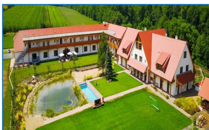
Photo 1 - overall view of the building
