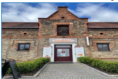
Photo 1 - overall view of the building
