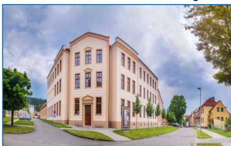
Photo 1 - overall view of the building
