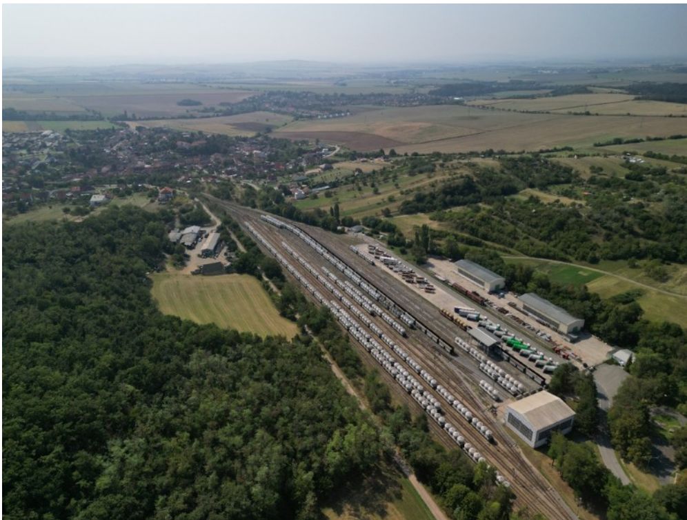
Figure2. Marshalling yard in the Cement Plant
