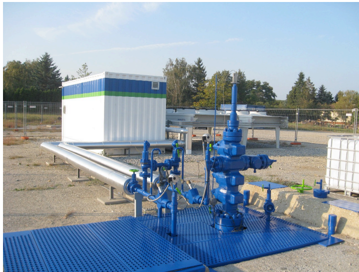
Figure C 6: Surface installation of the project Prottes T 11 with the geothermal container, eruptive cross and re cooler after repurposing (Bräuer, 2011).
