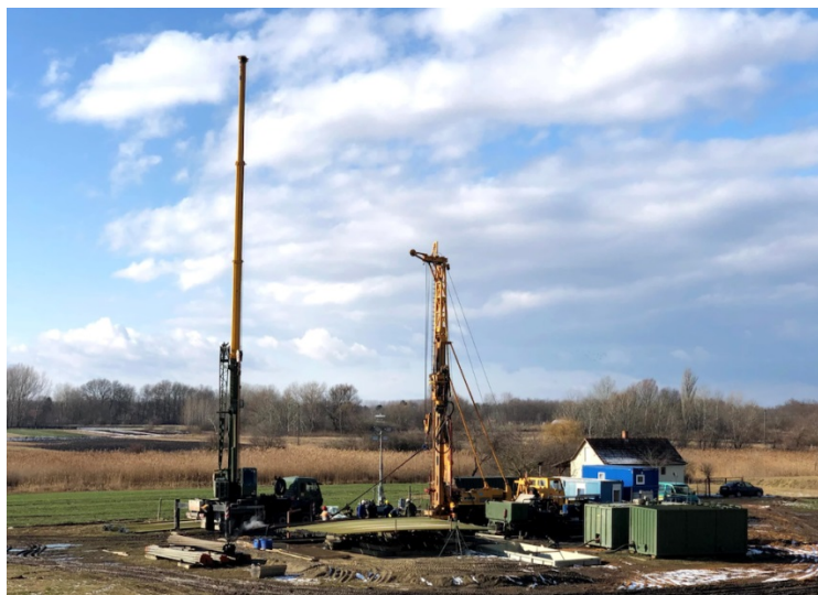
Figure C 10: Workover in Kiskunhalas ( https://www.thinkgeoenergy.com/first-closed-cycle-geothermal-heat-plant-set-up-in-hungary/ ).
