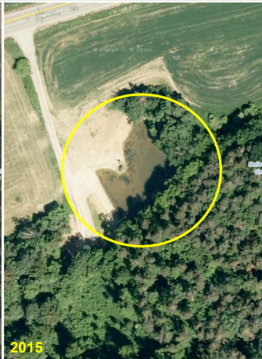
One year after restoration
