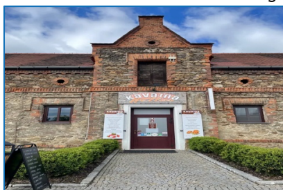
Photo 1 - overall view of the building
